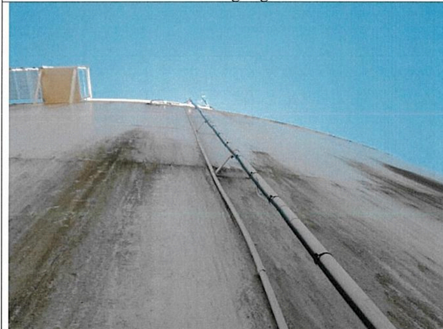
Varc gauge and conduit to roof
