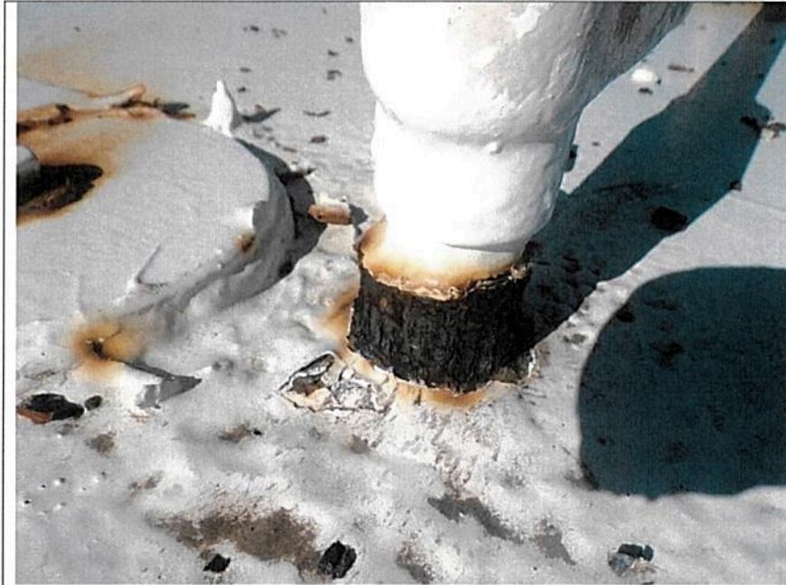
Corrosion at coupling attached to tank roof
