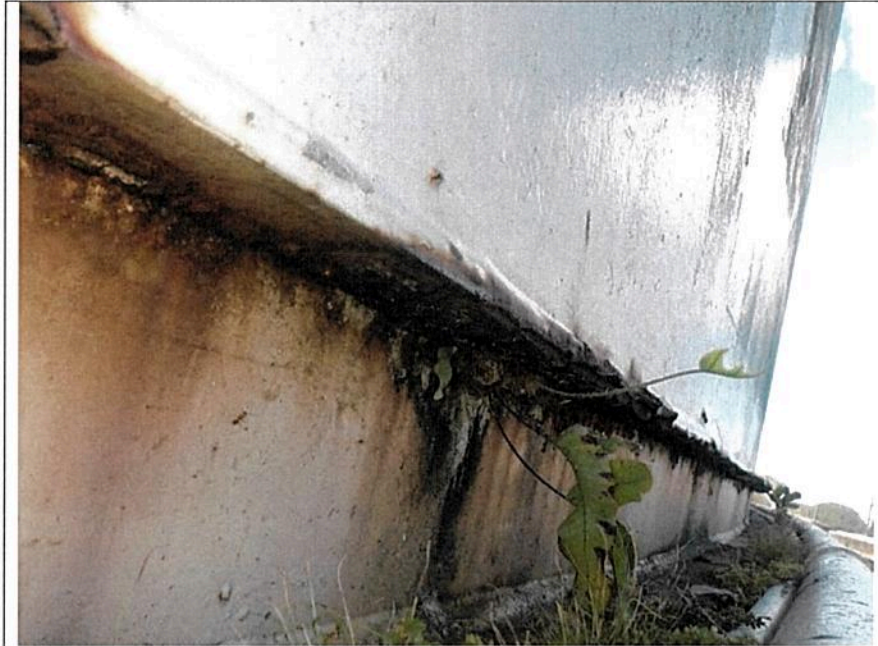
Corrosion on projection plate underside
