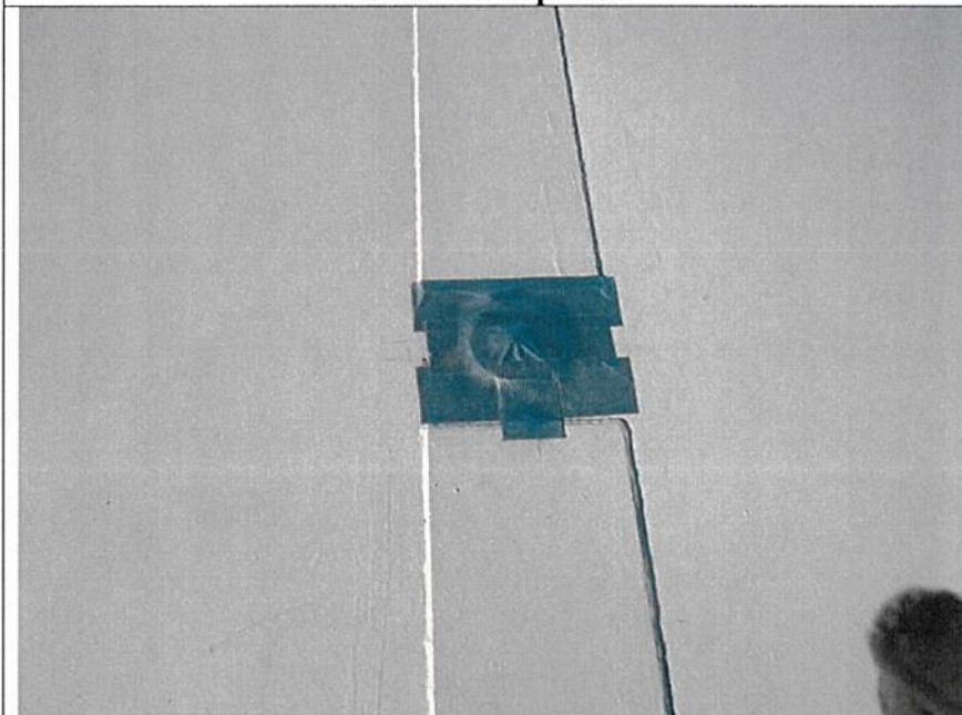
Tank roof with anode connection
