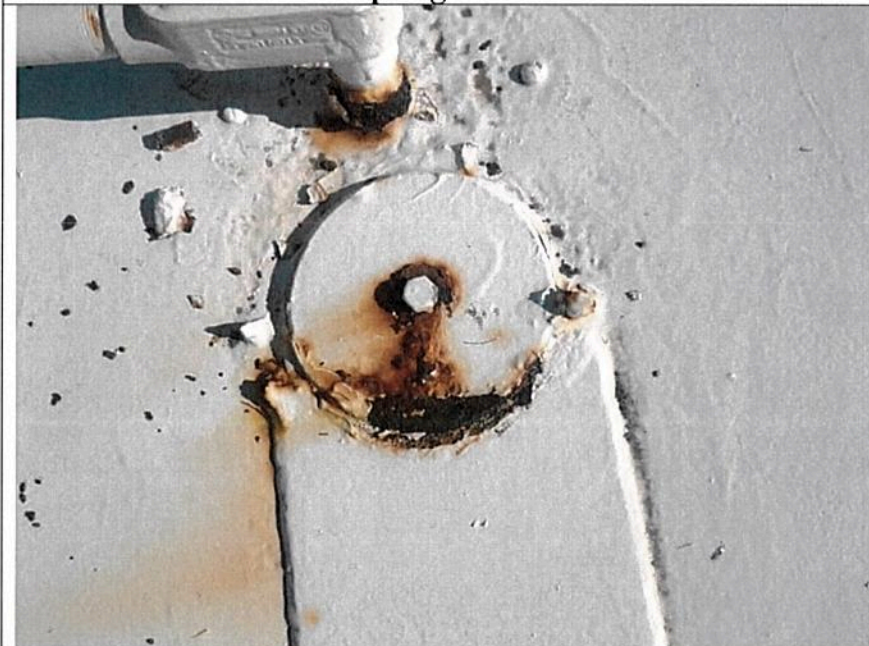
Corrosion at anode base
