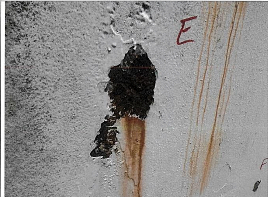
Shell corrosion
