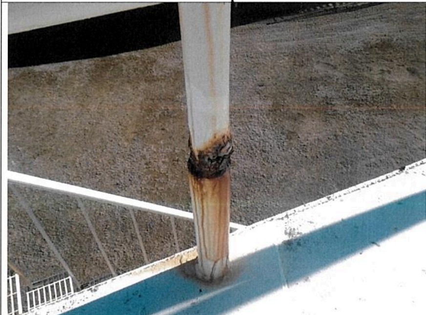
Corrosion at roof access
