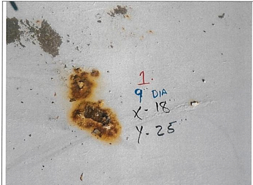
Area #1: 9" diameter area of corrosion
