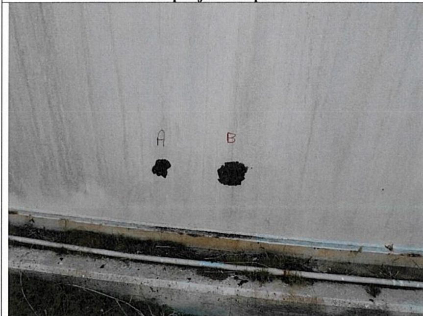
Shell corrosion
