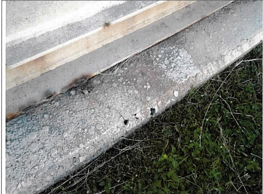
Concrete shrink cracking
