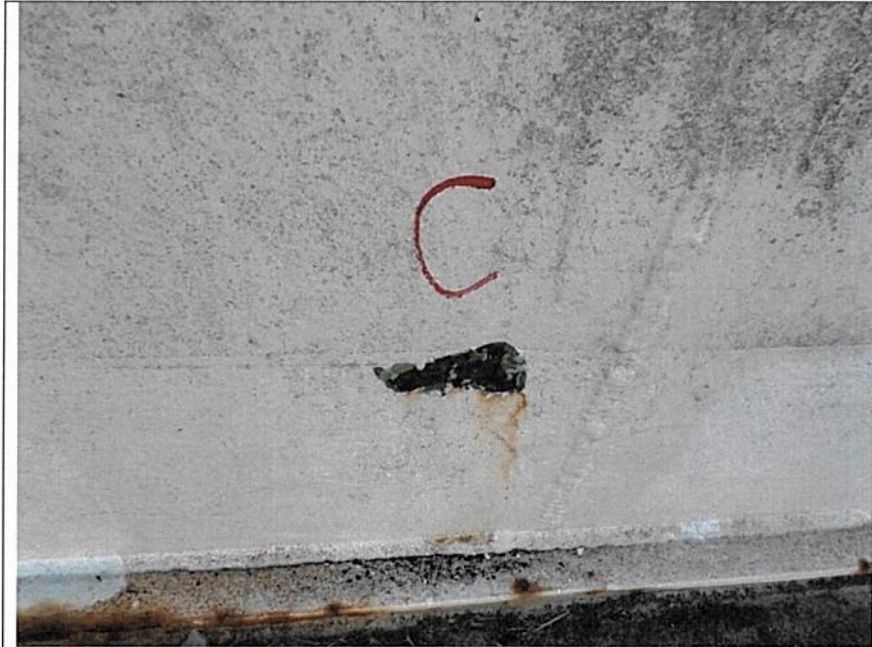
Shell corrosion
